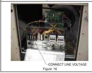
Ground unit with a suitable ground connection either through unit supply wiring or earth ground.
