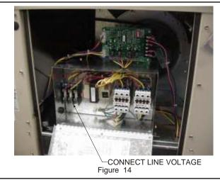
13. Ground unit with a suitable ground connection either through unit supply wiring or earth ground.
