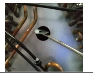
Figure 7. Remove T1 Sensor Knockout
